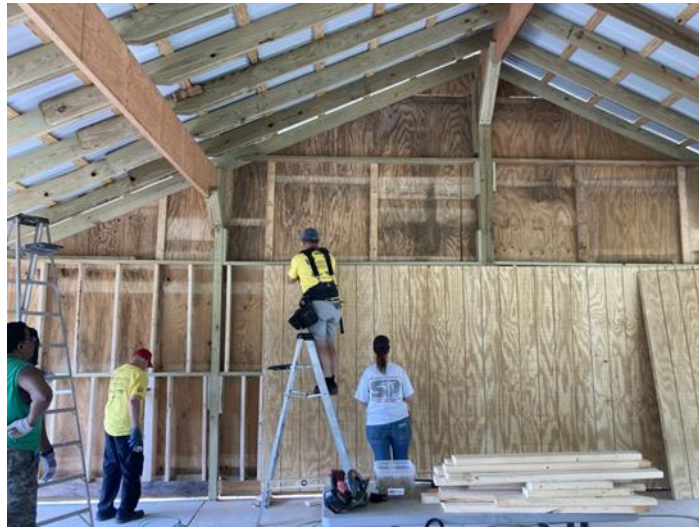
Building a wall – Arthur Ray, Bob Becker, Steve & Samantha Poole
